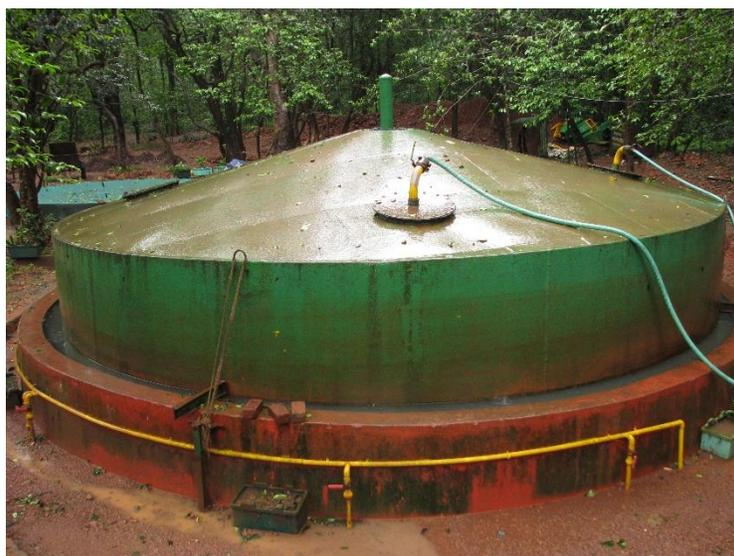
**Figure 22. Floating Drum Digester**
