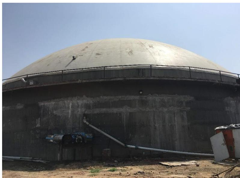
Figure 24. Completely Mixed Digester
