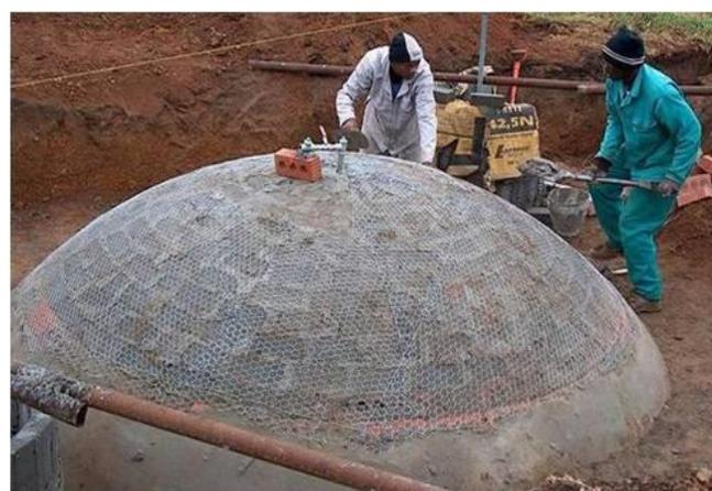
Figure 18. Fixed Dome Digester During Construction
